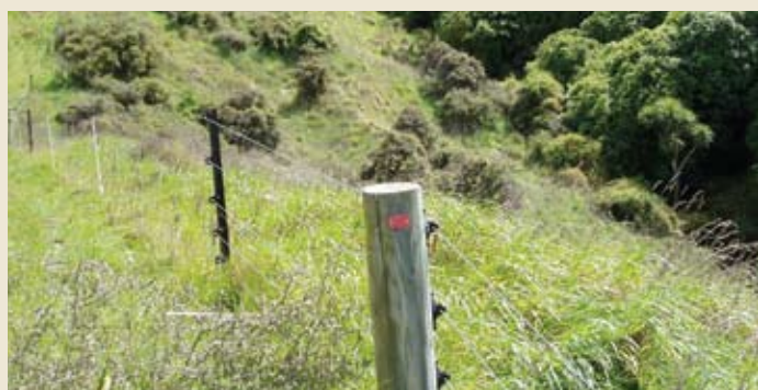
Hurunui shrubland and forest: 6-wire electric Y post fence with fibreglass droppers.
