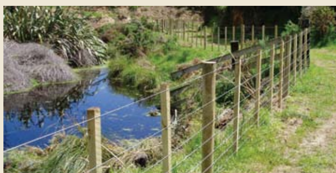
Kapiti Coast harakeke wetland: 7-wire post and batten fence.
