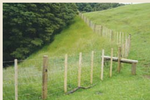
Franklin kauri-broadleaved forest: 8-wire (1 electric) post and batten fence.
