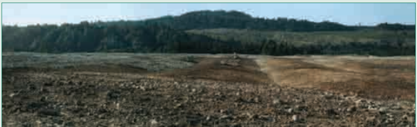
Humping and hollowing, October 2003; breaking up the ironstone pans and bringing subsoil material to the surface.
